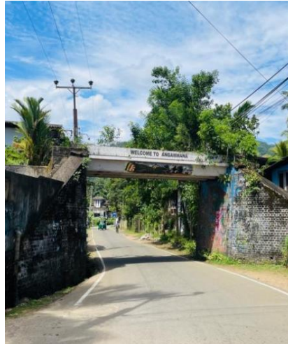
Figure 1 The Road leading to the Angammana village in Ratnapura. Photo by the author (2025).
